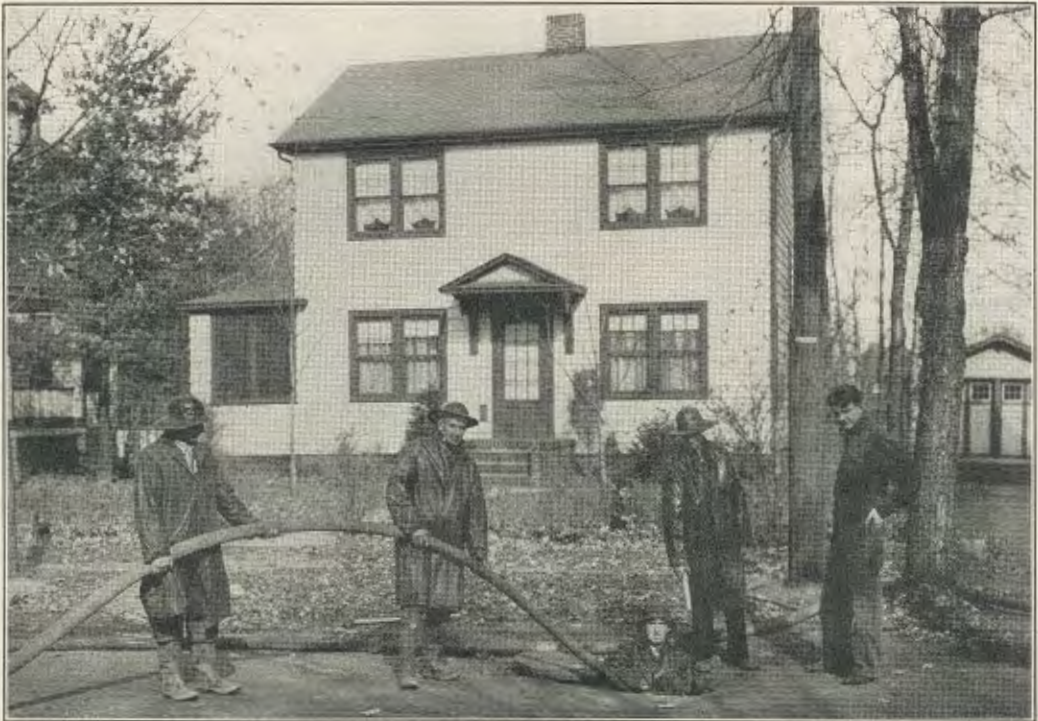
Sewer Flushing. (See last paragraph on Page 11.)
