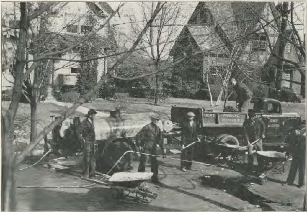
Asphalt Emulsion Treatment for Patching and Surfacing Bituminous Roads
