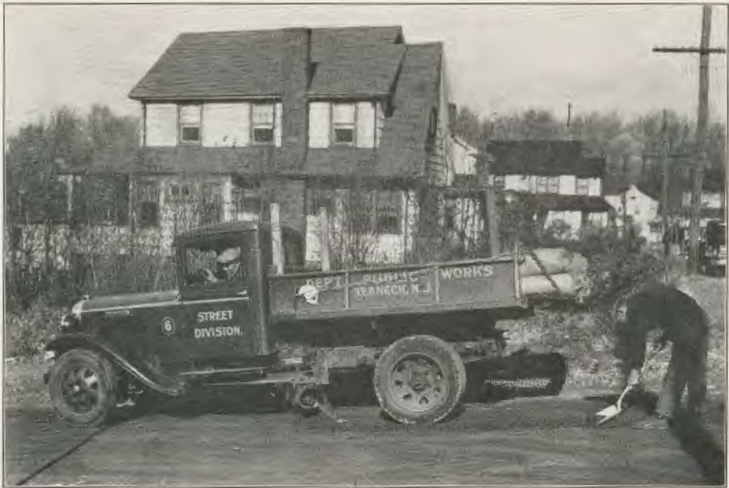
Scraping and Shaping an Unpaved Road by Means of Spring Type Grader Hooked-up to Truck
