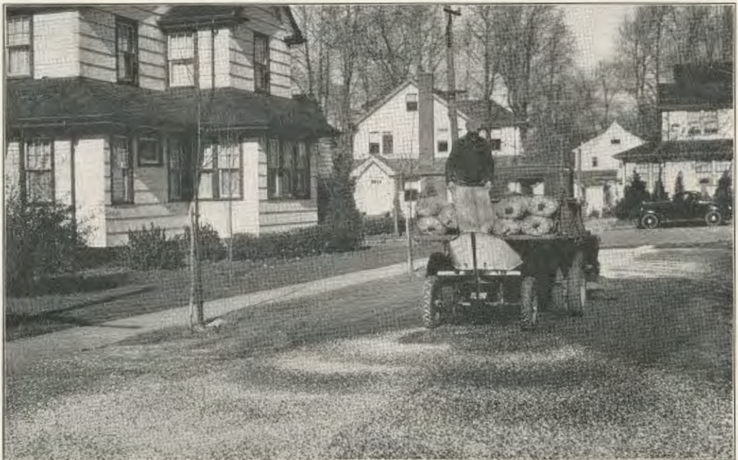
Spreading Calcium Chloride on an Unpaved Road (See third paragraph on Page 6.)
