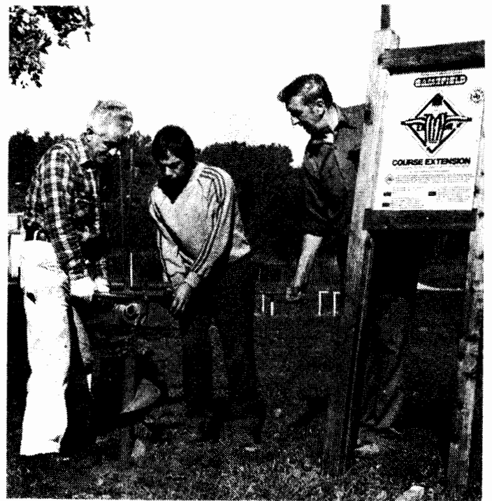
Department of Public Works employees are shown installing one of the signs that identify the new physical-fitness course for joggers and for walkers in Votee Park. There are a total of 20 activities, located at five locations in clusters of four each, throughout the park. The equipment was provided by the Township, with grants of $5,000 each from the Hackensack Health and Hospital Foundation and the National Fitness Campaign sponsored by the Wells Fargo Bank. The Township's cost, exclusive of DPW labor, was $5,450.
