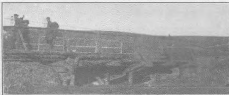
CO. "C" BRIDGE ACROSS THE AGRON RIVER
