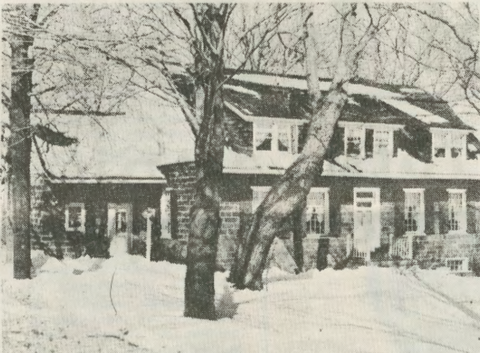
THE BRINKERHOFF-DEMAREST homestead on Teaneck Road is another classic example of "Jersey Dutch" architecture. It has been occupied continuously by members of the family since it was built in 1728.
