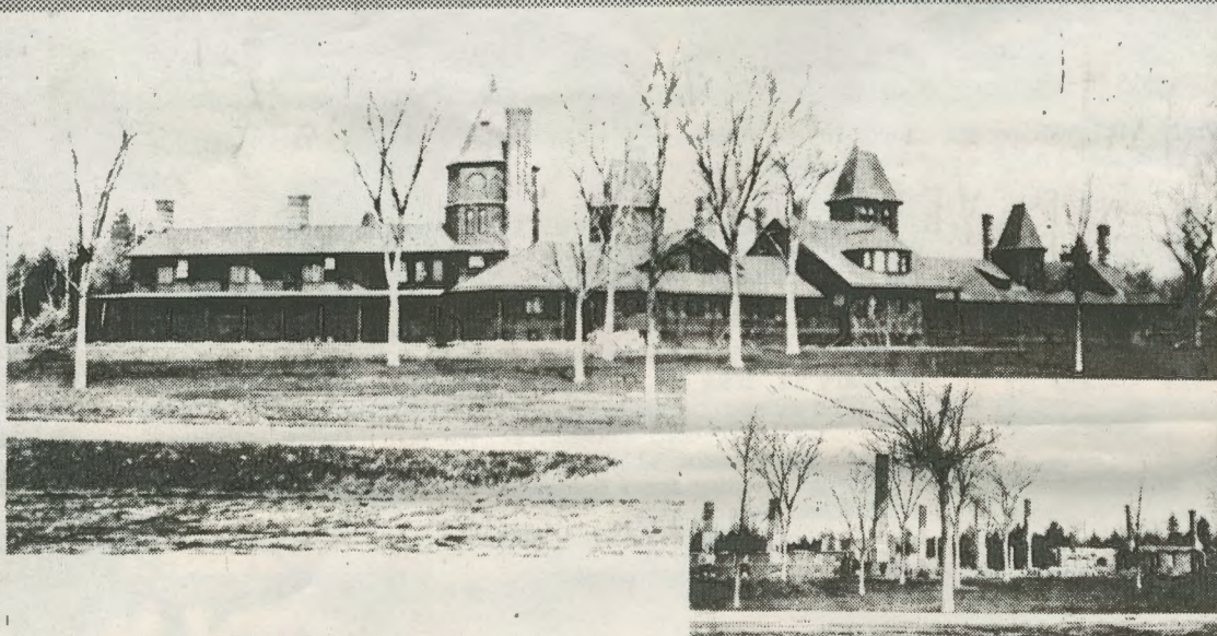
THE WILLIAM WALTER PHELPS MANSION, known as The Grange, stood on this beautiful estate from 1865 to 1889, when it was destroyed by a fire which left only the massive chimneys standing (inset). Teaneck's Municipal Building now occupies the site of The Grange. In his lifetime, Phelps is reputed to have planted over 500,000 trees in this area. Some of them still stand.
